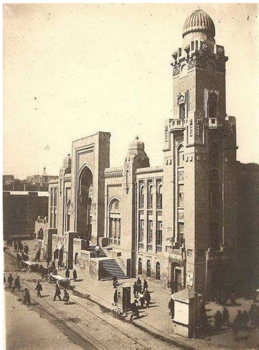
Railway station of Baku (1912) – architect Nicolay Baev
