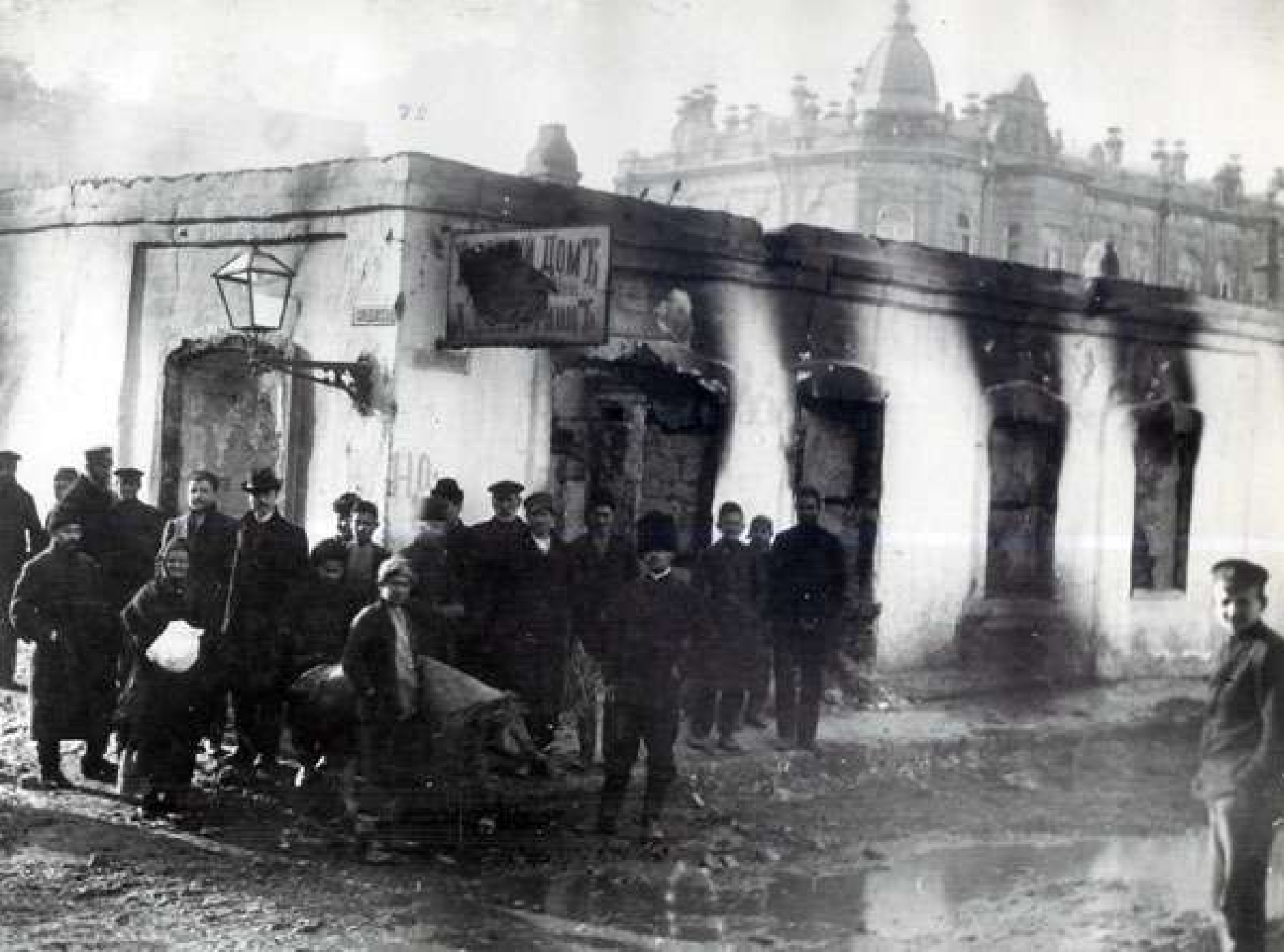
During the pogroms Tatars demolished the Armenian cultural sites, as well as houses and shops owned by Armenians. The burnt-down building shown in the photograph used to be owned by Armenians and was set to fire during the pogroms. The original photo is kept in the Fund of The Armenian Genocide Museum-Institute.
